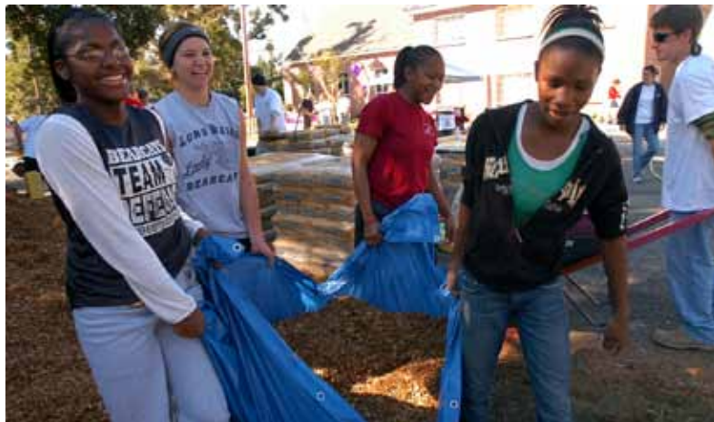
VOLUNTEERS HELP TO BUILD A KABOOM! PLAYGROUND IN NEW ORLEANS, LA. PHOTOS | COURTESY OF KABOOM!
